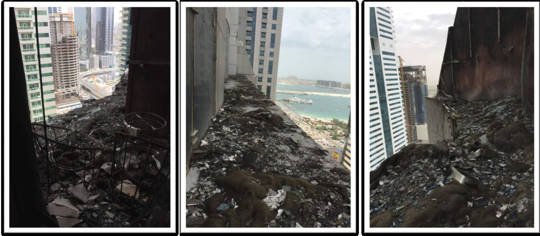
Burning Debris fell onto 30 th Floor Balcony
