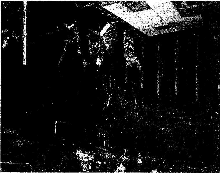
Looking from north door of Zebra Room at wall of hallway opposite Zebra Room. Note combustible finish materials. NFPA
