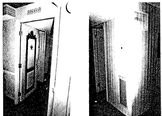
From corridor looking into guest room, fan-coil unit within room took make-up air from corridor through air inlet above door. Fan-coil unit in room delivered air to room (air outlet at top) taking make-up air from corridor and recirculating room air thru air inlet at bottom. (Credit: NFPA)
